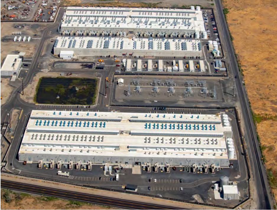
Amazon Web Services (AWS) data center in the US (Credit: Tedder)
